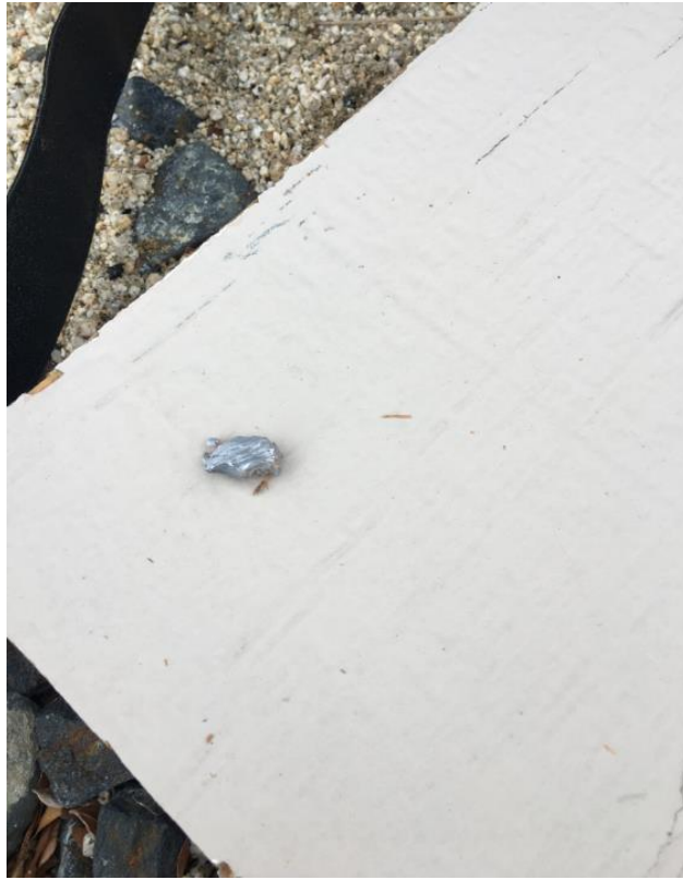
Photo: recovered bullet fragment from exterior wall of apartment
